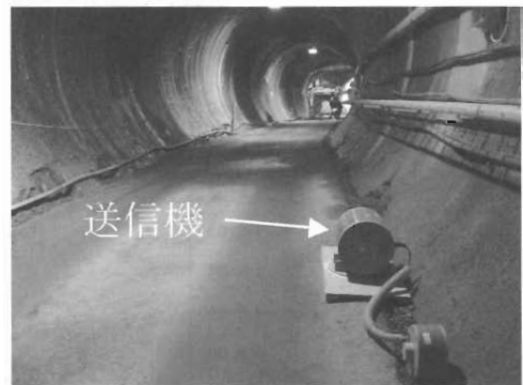
Fig.32 Experiment in Underground Laboratory of SKB
