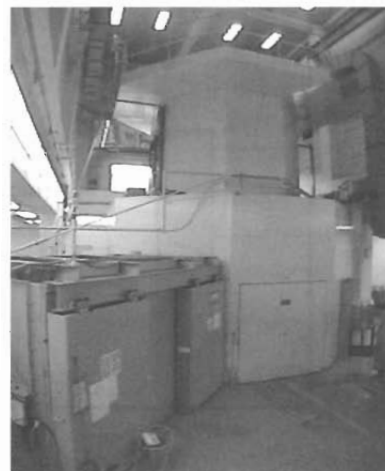
Fig.18 Remaining Rikkyo University Reactor
