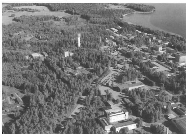
Photo 1 Site of Studsvik RadWaste
