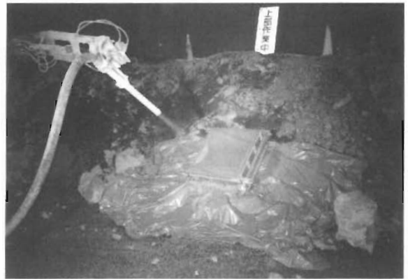
Fig.20 Bentonite Barriers by Spraying Methods
